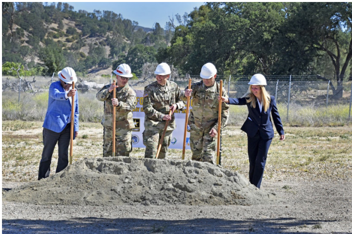
Groundbreaking for microgrid project, Fort Hunter Liggett, CA.
